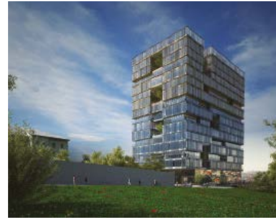
Central and eastern Europe: The 30-storey Now Bomonti building by Tabanlıoğlu Architects, currently under construction in Istanbul.
